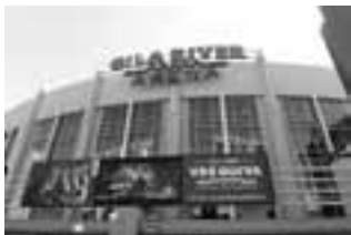
Gila River Arena
